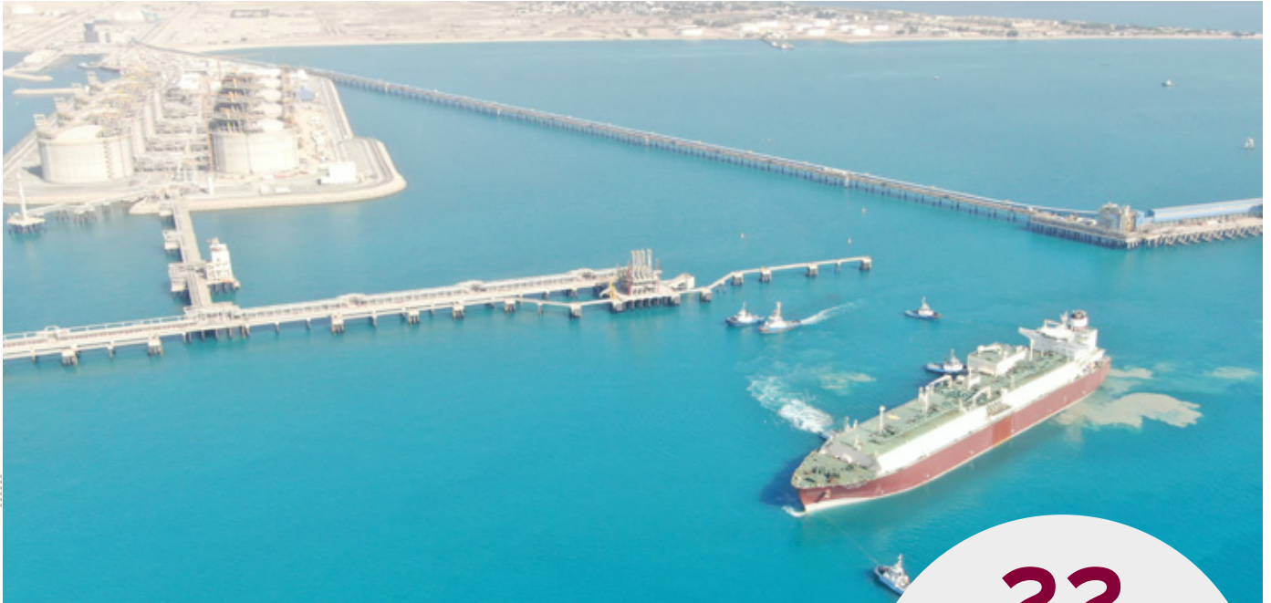
The cargo was loaded aboard the Qatargas-chartered LNG vessel, 'Al Kharsaah', at Ras Laffan on 9 July 2021 and delivered to Al-Zour LNG terminal, owned and operated by Kuwait Petroleum Corporation (KPC), three days later.
