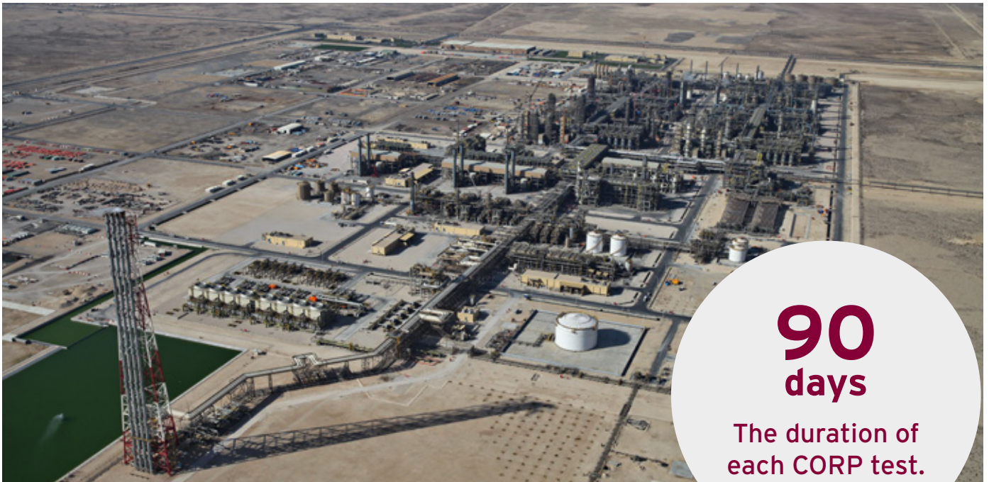
Barzan consists of three offshore wellheads and two pipelines feeding two gas processing trains. Each is sized at 950 million cubic feet/day of Full Well Stream (FWS), representing an important element of Qatar's energy infrastructure.
