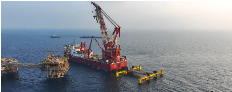
Pile Installation CP6s jacket.
