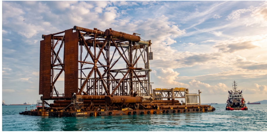
A key milestone was the delivery of the WHPI3N Jacket, fabricated at the QFAB Yard and executed by McDermott.
