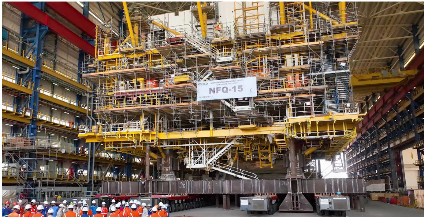
The NFQ15 topside (Wellhead Platform) for the NFXP project was assembled in the QFAB Yard under the 'Design One, Build Many' philosophy to drive standardisation, efficiency, and cost optimisation.
