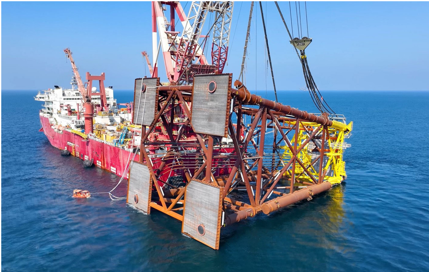
Offshore installation of the LQ6S jacket.
