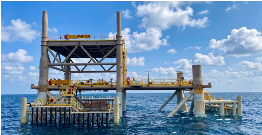
Weighing more than 2,800 tonnes, WHP12N represents the first offshore jacket fully fabricated in Qatar, marking a new era of local engineering for the North Field.
