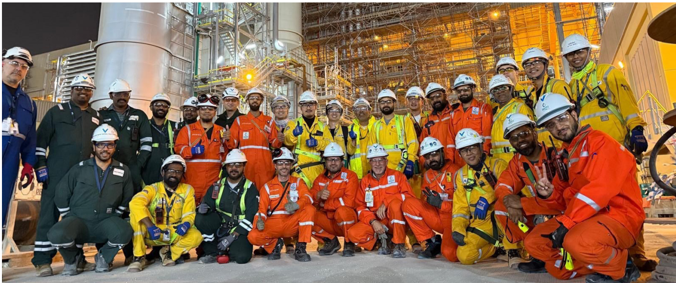
The solo run test was jointly executed by CTJV and Baker Hughes, with support from QatarEnergy LNG Project Management Team (PMT) Subject Matter Experts (SMEs) and Operations Expansion and Startup (OES).
