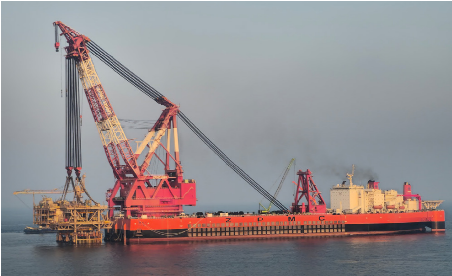
The three new NFPS riser platform topsides RP6S, RP4S and RP7S were successfully installed in late December 2024 using the heavy-lift vessel ‘Zhen Hua 30’.
