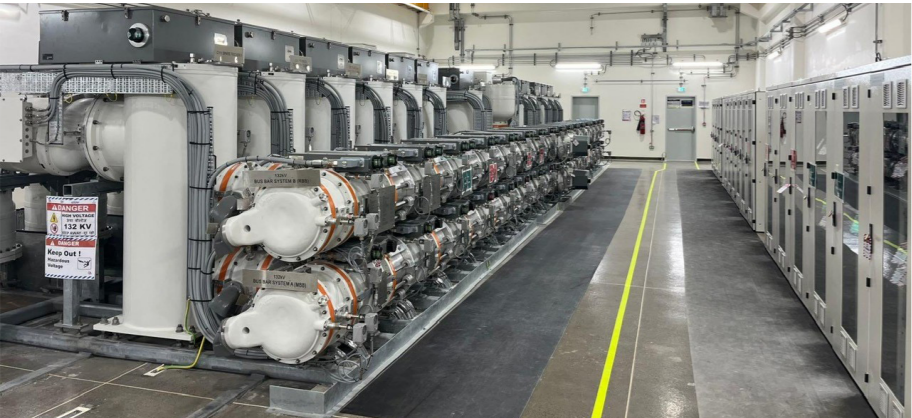
The 132kV switchgear energised.
