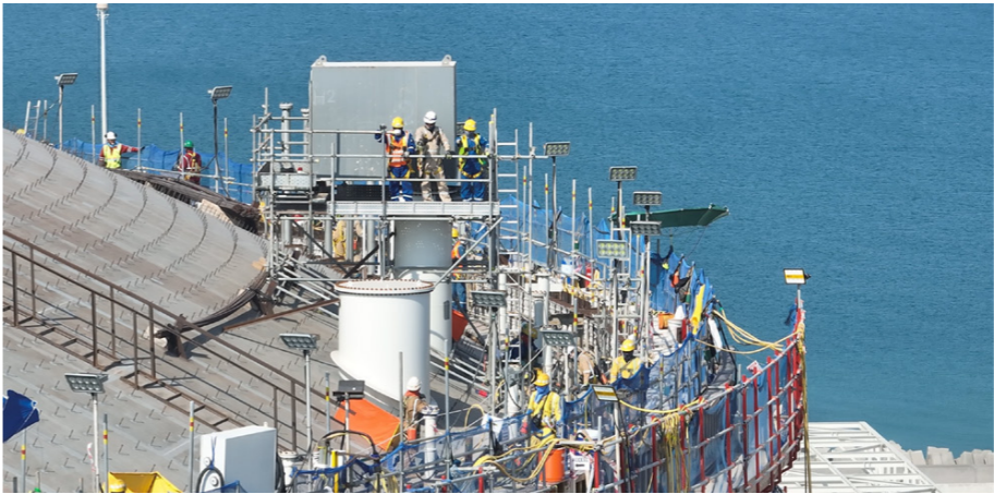
The roof raising 47T-7101 lasted approximately 2.5 hours. The roof weighs 950 tonnes and measures 86 metres in diameter.
