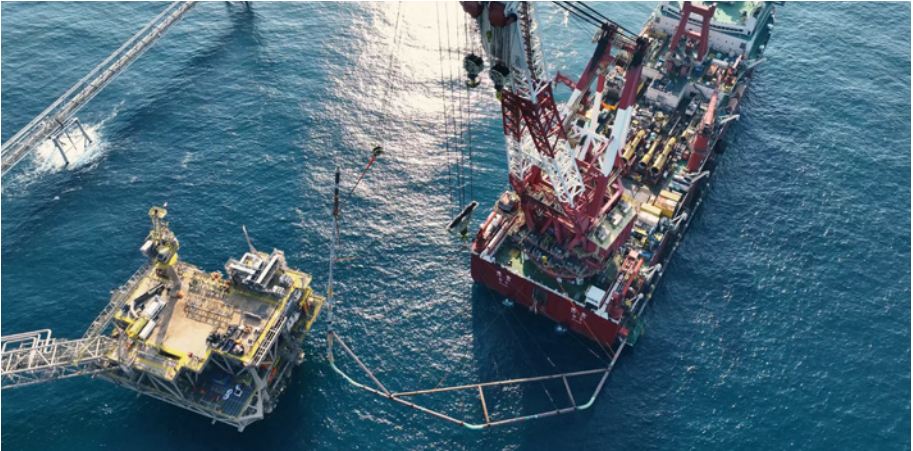
The dynamic position method reduced average installation time per riser from 12 days to just five days.
