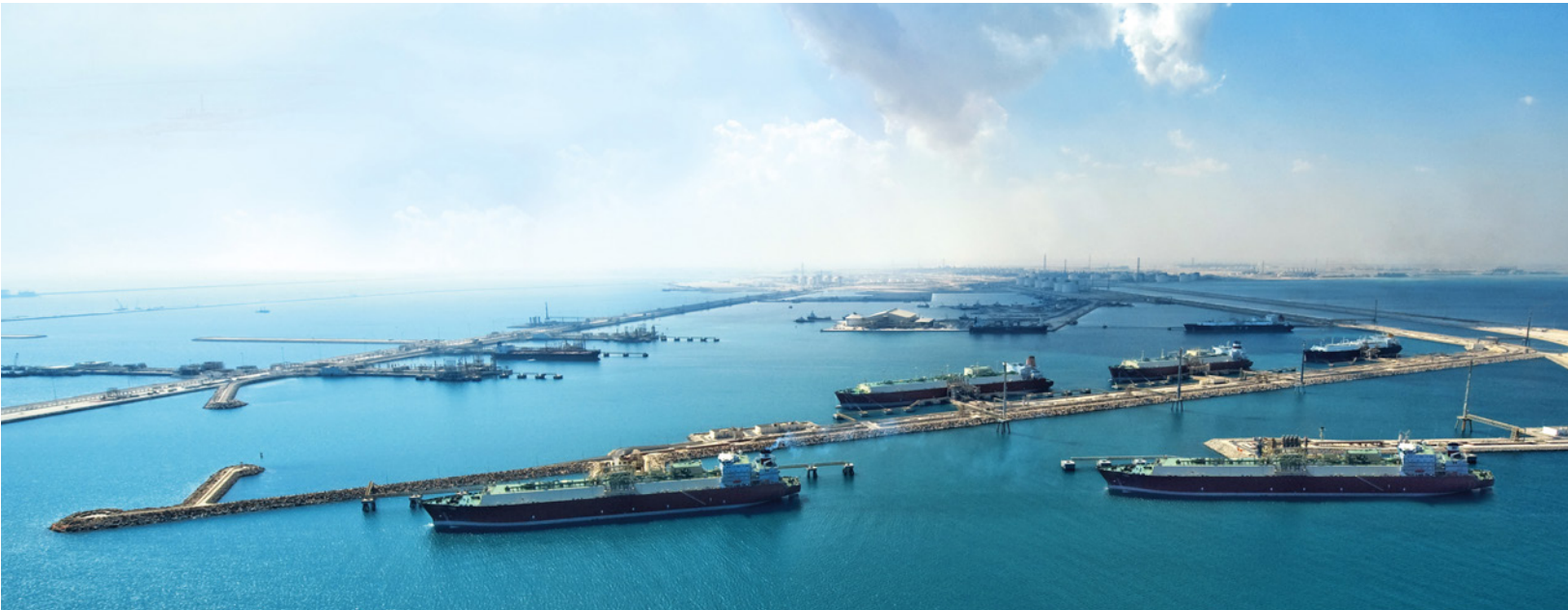
JBOG: 10 years, 17 million tonnes of GHG emissions saved, 60% flaring reduction.
