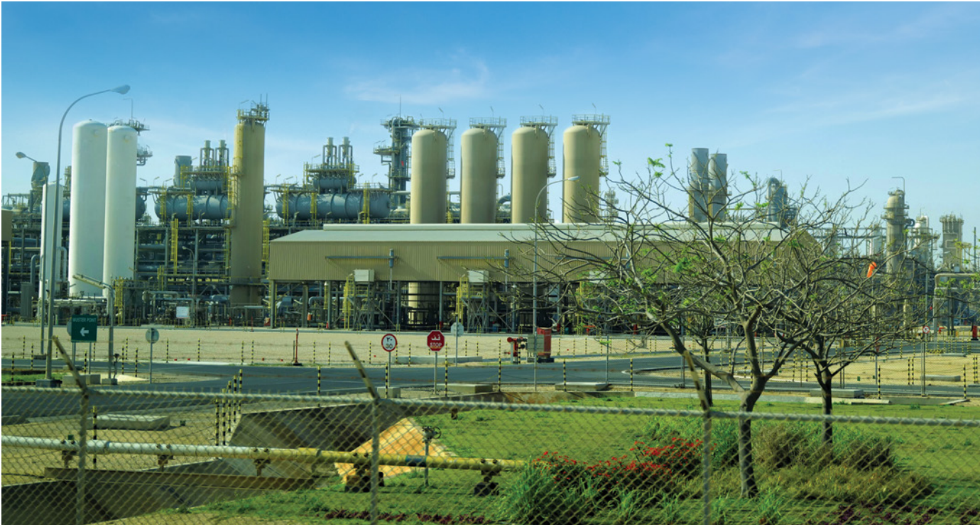
Barzan Gas Plant: Powering Qatar’s growth and meeting rising energy demands.
