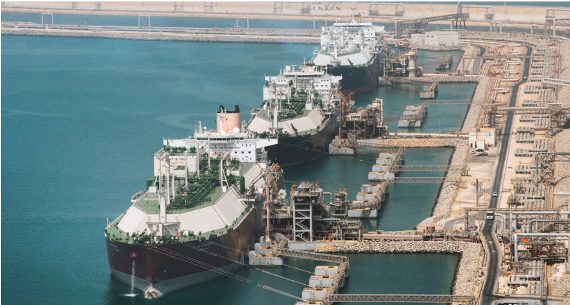
Launched in 2006, Ras Laffan Terminal Operations (RLTO) was designed to streamline storage and loading.
